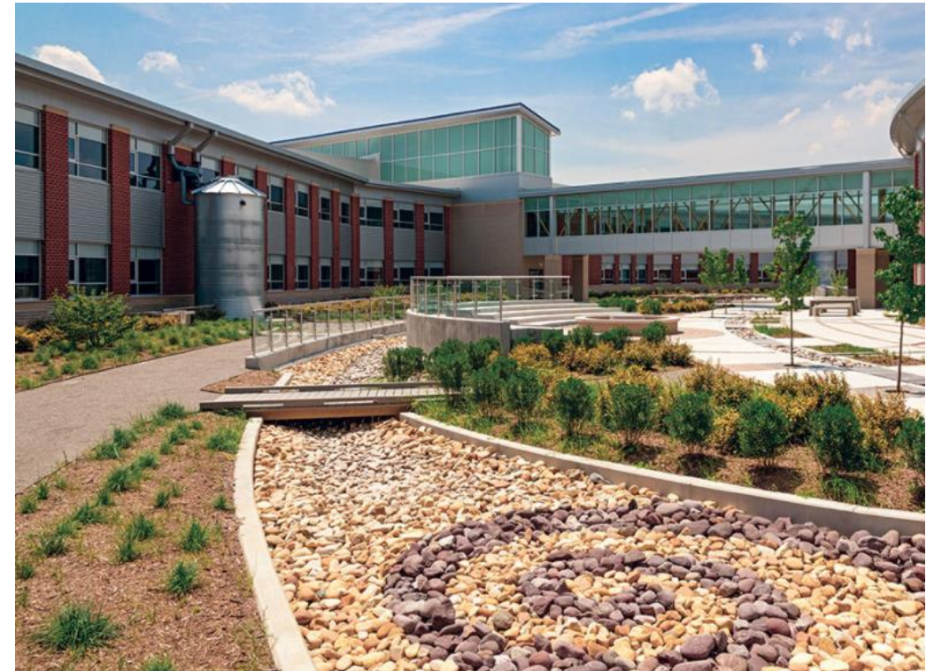
Virginia Beach Public Schools – Floyd E. Kellam High School in Virginia Beach Rainwater from hardscape directed to planted and decorative swales for infiltration on site http://plus.usgbc.org/building-curriculum/
