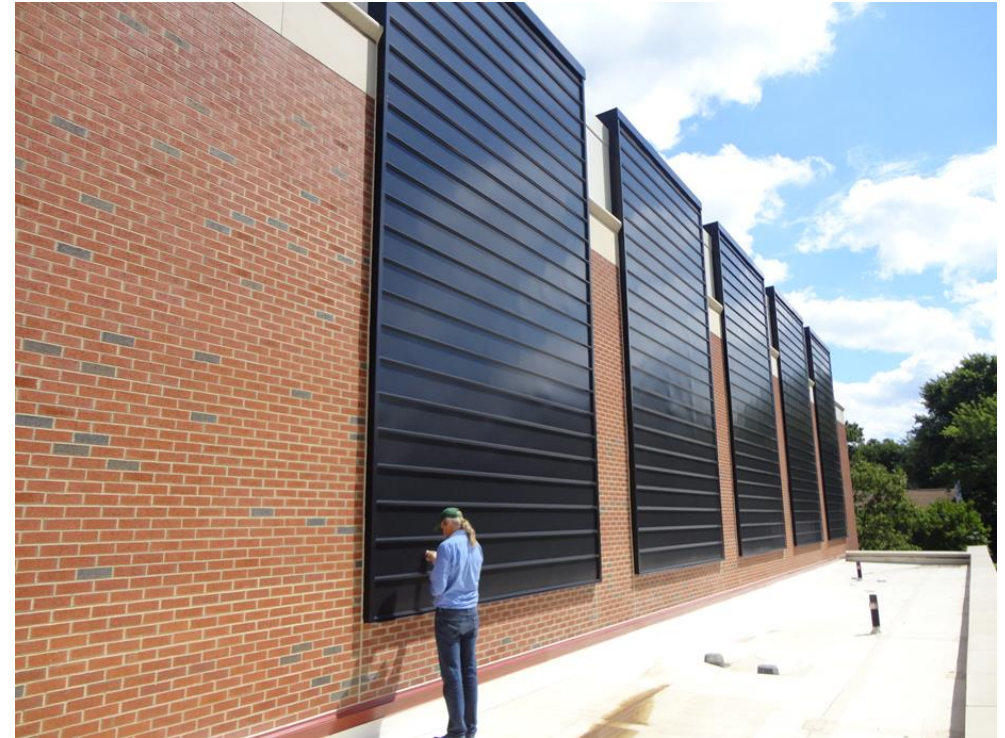
Solar Wall – image courtesy of http://www.taitem.com/news/lou-cherry-road-solar-wall-1/
